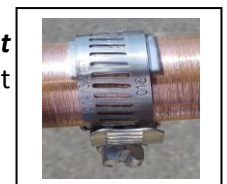
FIGURE 6. CLAMP TIGHTENED
